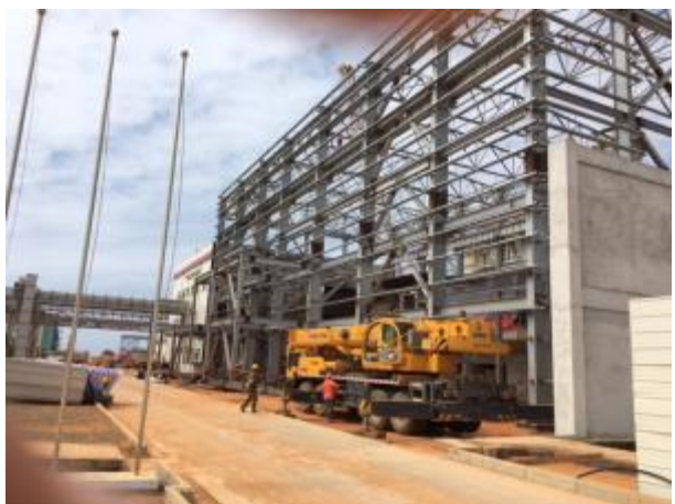
Steam turbine building
